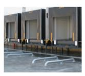
**Truck guides** The guides protect the facility, as the truck is aligned to make it easier for it to enter the bay.
