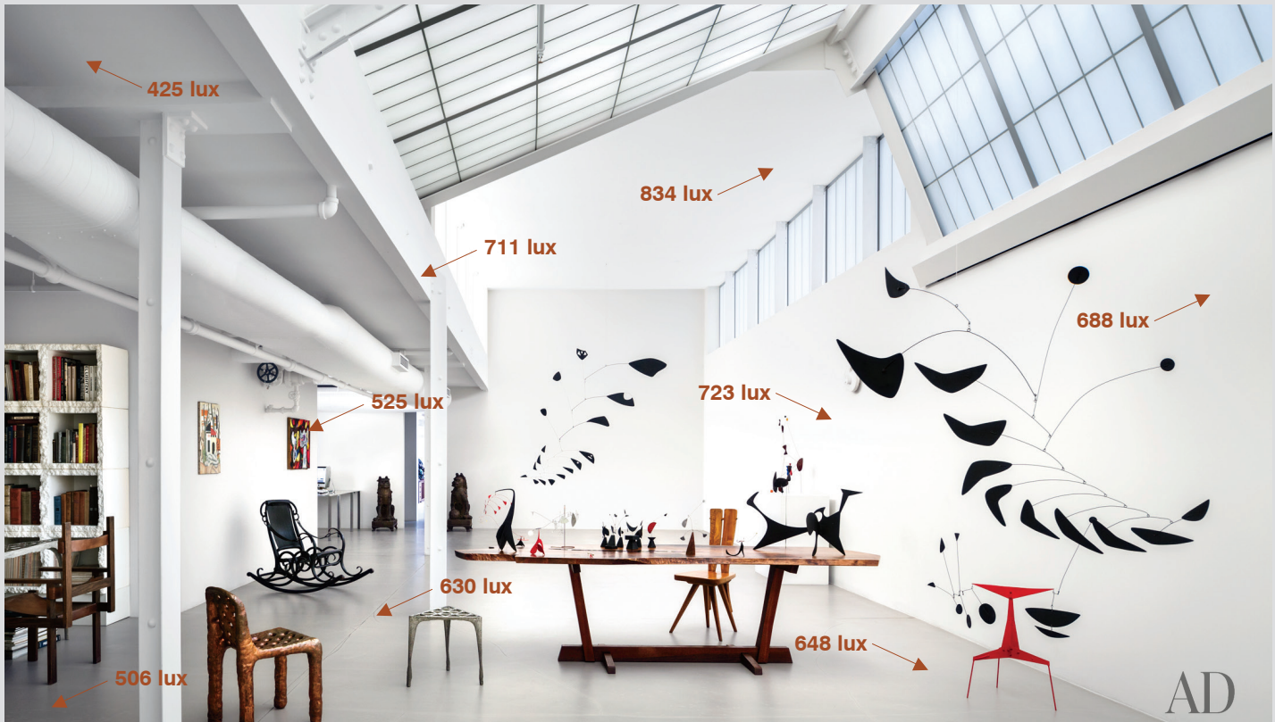
Calder Foundation | New York, NY | Stephanie Goto | Custom Skyroof and Wall System
