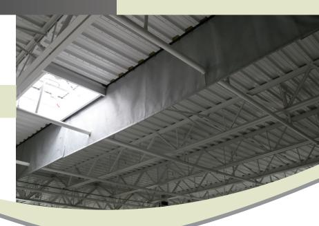
**Description.** SG Draft is a code-compliant, lightweight, fixed fabric curtain, semi-permanent or temporary, system for large vertical openings. The SG Draft SGTex10 smoke curtain material is a glass filament fabric with a glass fiber material on one side.
